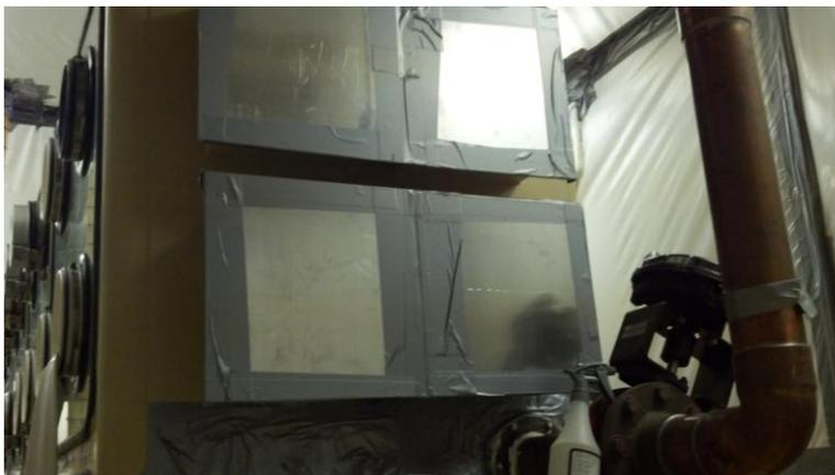
Figure 2: Ventilation ports after plenum removal
