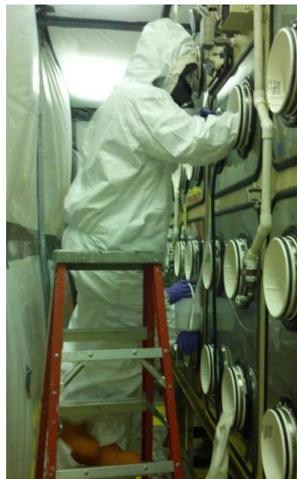
**Figure 1: Workers spraying fixative in the glovebox**
