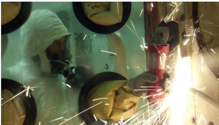
**Figure 4: Grinding Seized Bolt Heads to Remove Transfer Port**
