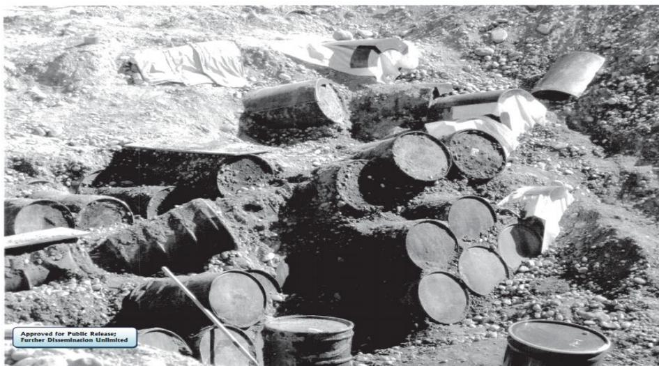
Figure 4. Drums and debris uncovered in a trench of the 200 East Area burial ground. The configuration of the drums necessitates manual excavation and handling.
